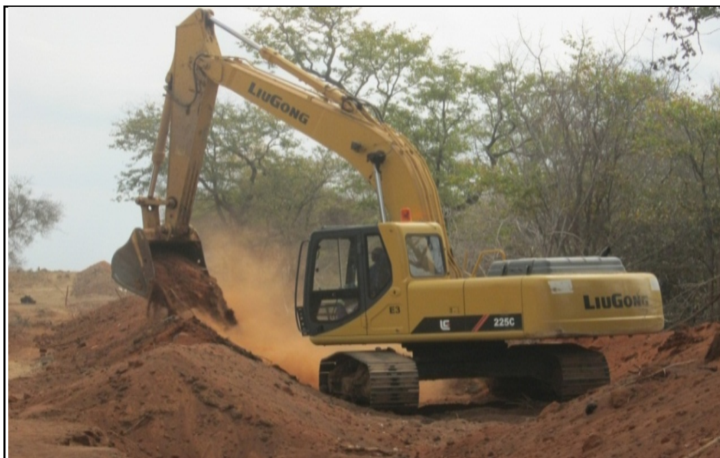
Figure 3. Land and bush clearing operation.
