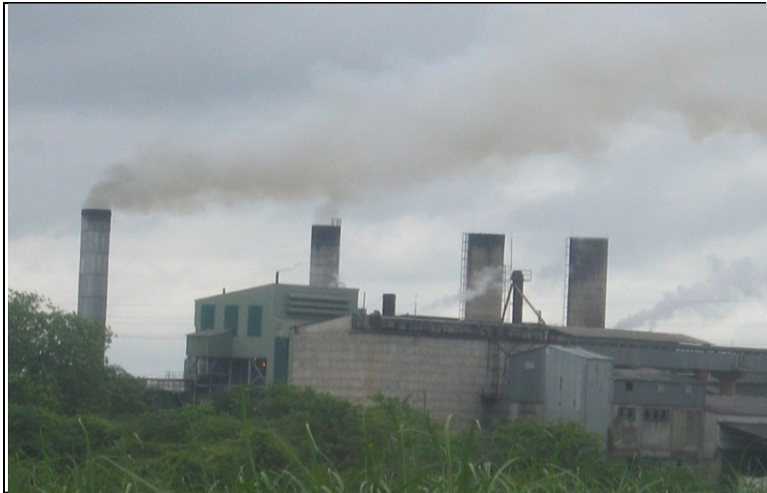
Figure 1. Air pollution due to boiler stack emissions.
