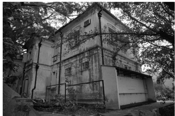
Figure 15. Old Tai-O Police Station (Chung 2012).
