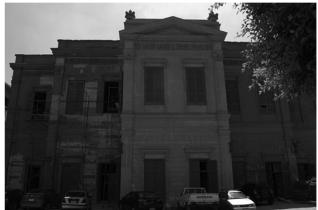
Figure 20. Exterior façade of Ismail El-Mufatesh Palace (Abdelmeguid 2016).
