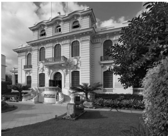
Figure 9. Exterior facade of ANM (Goddio 2019).
