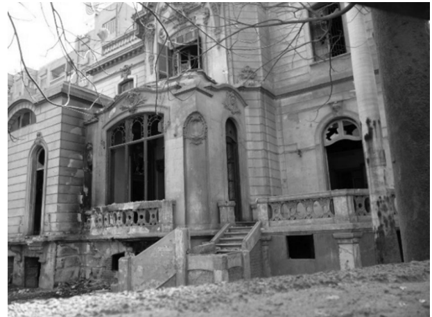
Figure 5. Villa Casdagli in Cairo, Egypt after fire damaged the façade (Pathan 2013).
