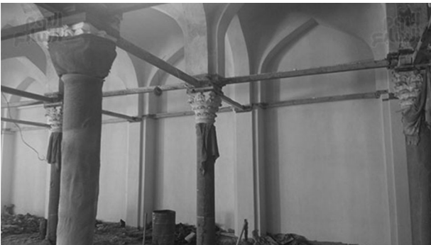
Figure 21. Inside Zaghoul Mosque, showing restoration of columns (Mansour 2018).
