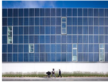
Figure (3) SunPower Equinox Photovoltaic Building Facades
