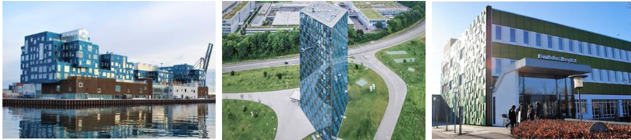
Figure (4) Kromatix Solar Photovoltaic Building Facades
